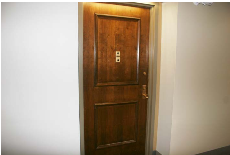
PHOTO #24 All unit doors will be retained in the corridor refurbishment project, but will be carefully re-finished.
