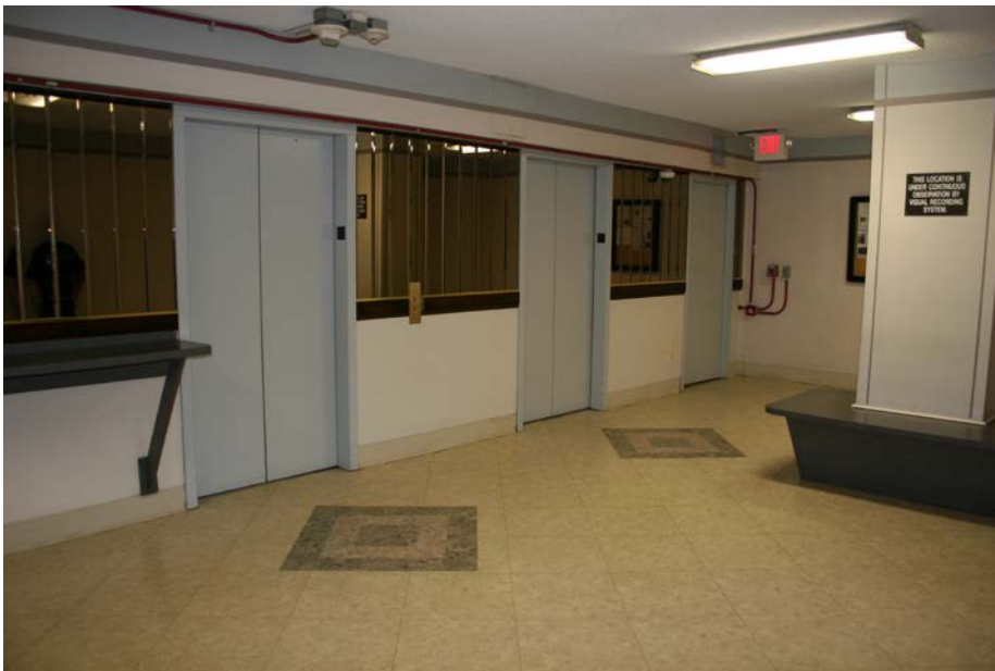
PHOTO #23 The garage elevator lobbies and the service lobbies will also be upgraded near-term.
