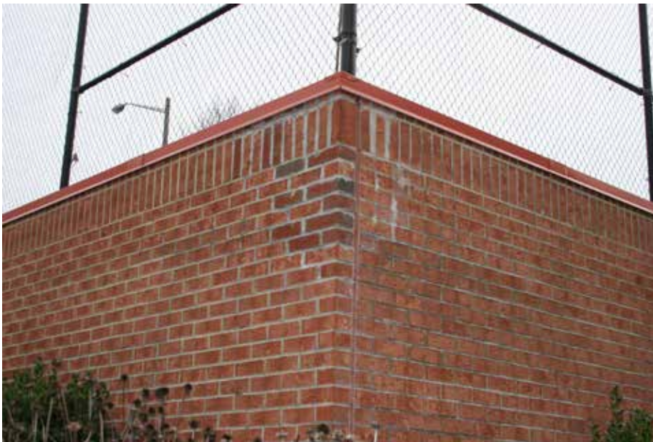
PHOTO #22 The 2007 recommended engineered repairs to the masonry retaining wall appear to have been successful.
